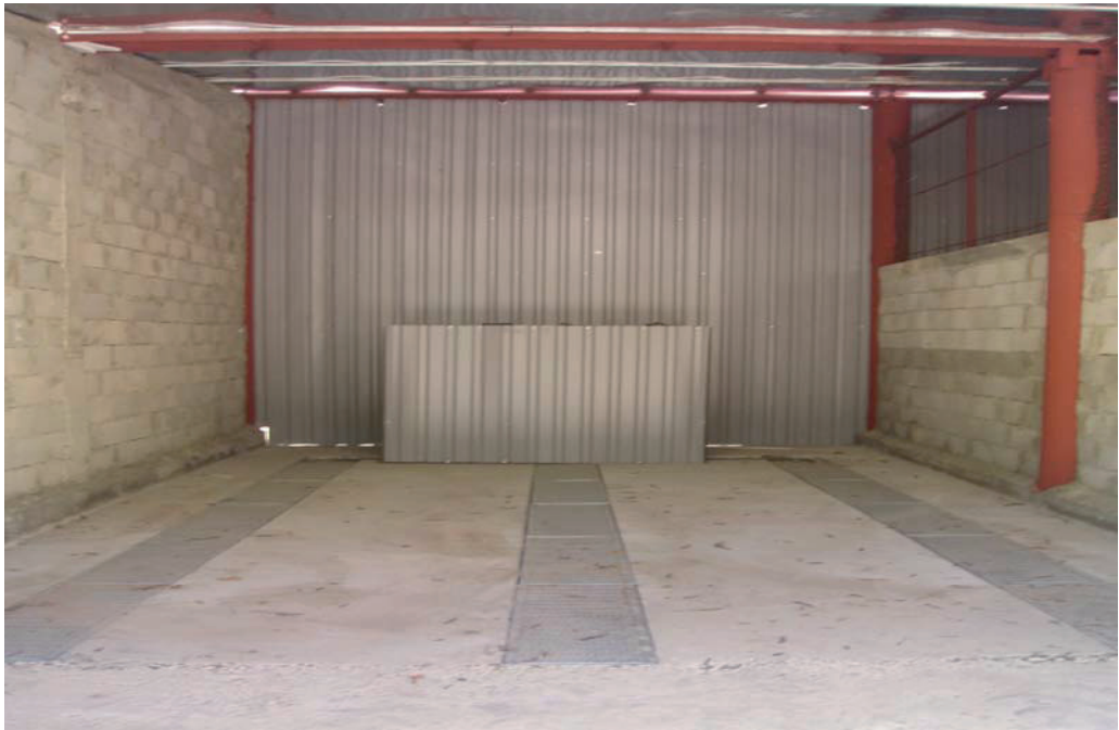
Figure 7: Internal space of one drying section with air divider and floor channels
