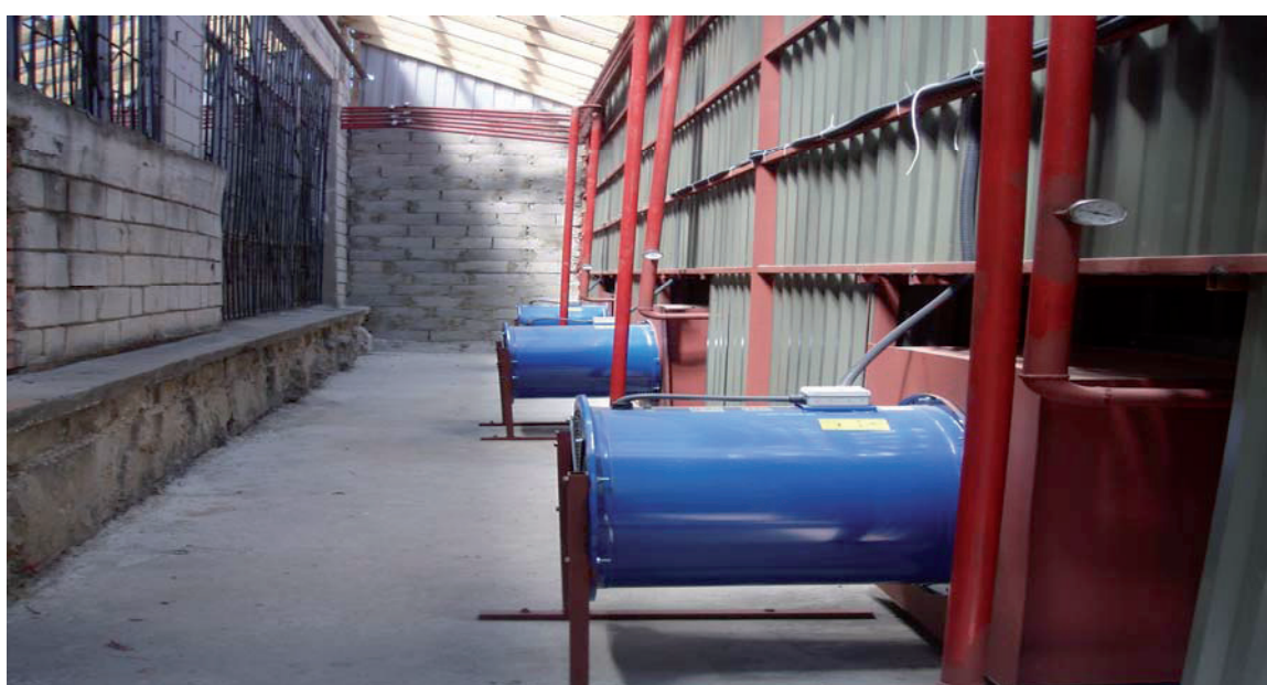
Figure 6: Placing fans with assembled heat exchangers
